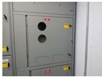
Service Entrance w/Metering – 15kV, 1200A, 50kA in PDC
